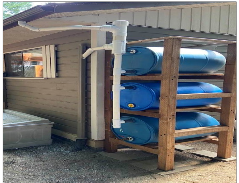
An example of a 3-barrel rainwater collection by a SPID resident.
